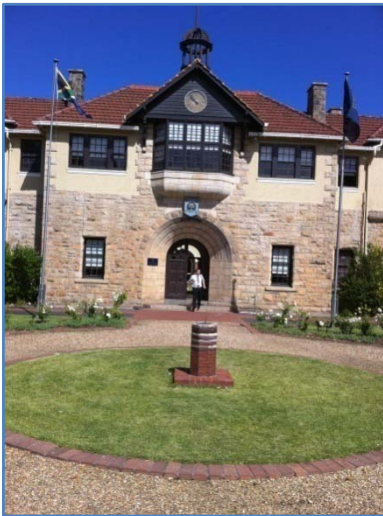
Rondabosch Primary School
